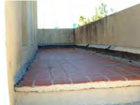
Photo of the red tile that lead to the north opening to the 3<sup>rd</sup> floor. In the far left corner a small tree had begun to grow out of the tile.
