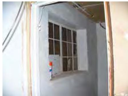
Basement window that had once been visible from the exterior of the building. There is approximately a foot of space between it and a cinderblock wall that encases the window.
