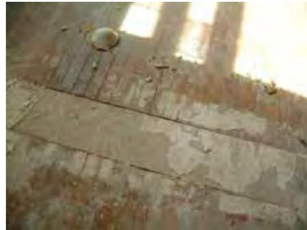
Section of flooring in the main lobby where a section had been patched where a stud wall had been removed.
