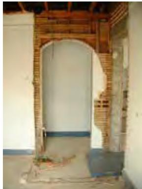
Arched doorway that used to lead to the basement stairs. The wall surrounding it features what is left of the plaster and slat walls that were original to the building.
