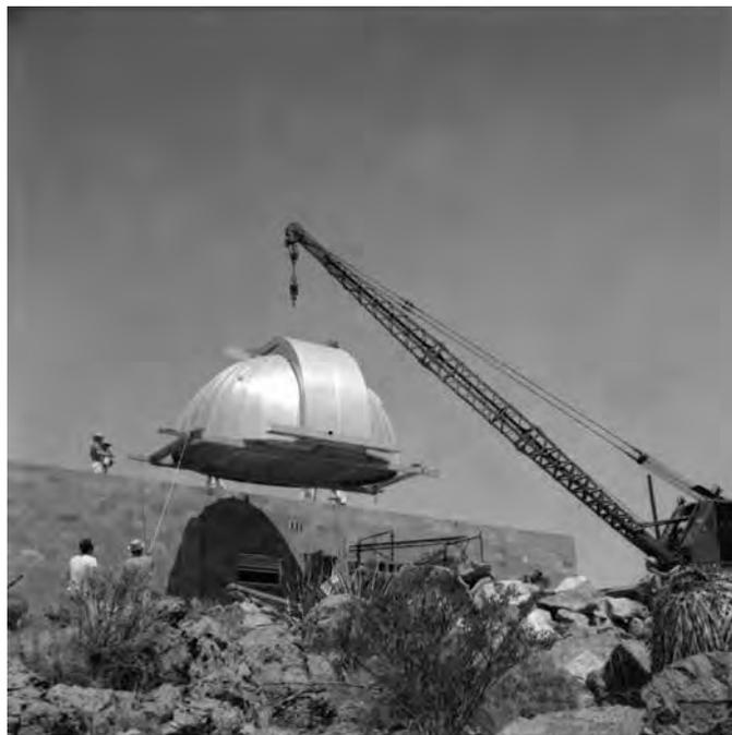
Lifting one of the domes onto the top of the building in 1964.
