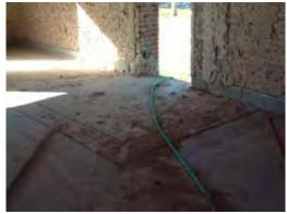
Original west entrance. The stairs that used to be here were filled in by concrete.
