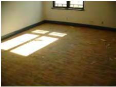
In a room in the north wing of the building, the hardwood flooring is covered in adhesive that used to secure flooring that had been laid over it.
