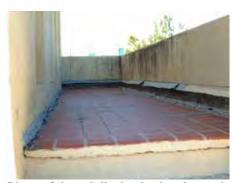
Photo of the red tile that lead to the north opening to the 3<sup>rd</sup> floor. In the far left corner a small tree had begun to grow out of the tile.
