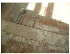
Section of flooring in the main lobby where a section had been patched where a stud wall had been removed.
