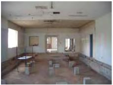
East wing of the building. The rectangular blocks of concrete are footings that supported the floor. The floor had also been laid over the original steps on the exterior of the building.
