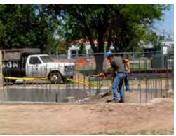
Digging the footing for the new elevator shaft.
