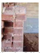
Section of the exterior wall of the dining hall. Shows the original brick with a coating of stucco.
