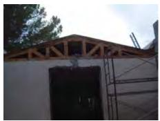
End of the west wing that has had a doorway punched through the exterior wall of the addition to allow passage to an additional addition to the west wing.
