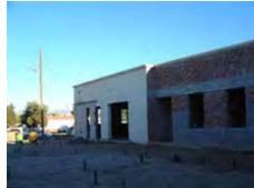
Soil has been built up to the level of the thresholds of the north entrances to the building to support the new addition.
