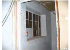
Basement window that had once been visible from the exterior of the building. There is approximately a foot of space between it and a cinderblock wall that encases the window.
