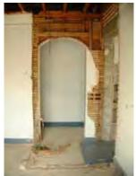
Arched doorway that used to lead to the basement stairs. The wall surrounding it features what is left of the plaster and slat walls that were original to the building.
