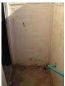
At the bottom of the exterior steps to the basement, there is evidence of an opening that had been filled in with cinderblock.
