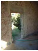
The original west Entrance. Cinder Block is visible where the door way was narrowed from two doors to one.
